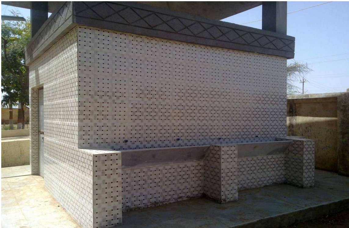
Ambikanagar Primary School-newly constructed drinking water facility.
