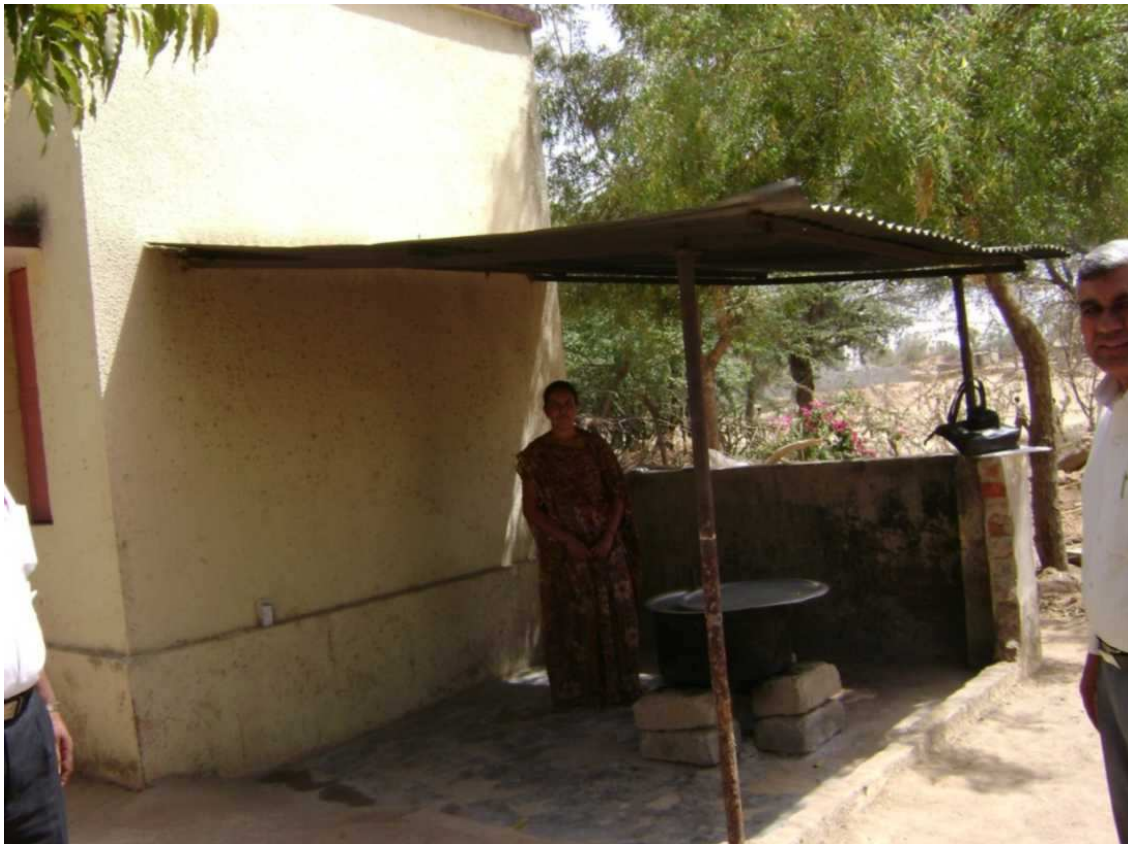
Lakhani Upper Primary School - MDM kitchen Facility-just a shed
